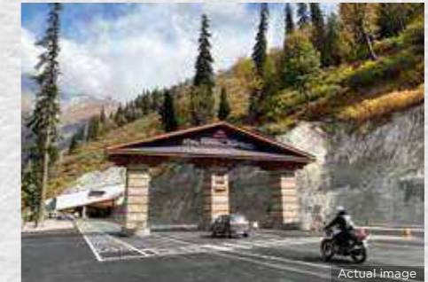
Atal Tunnel, Himachal Pradesh, 2020
